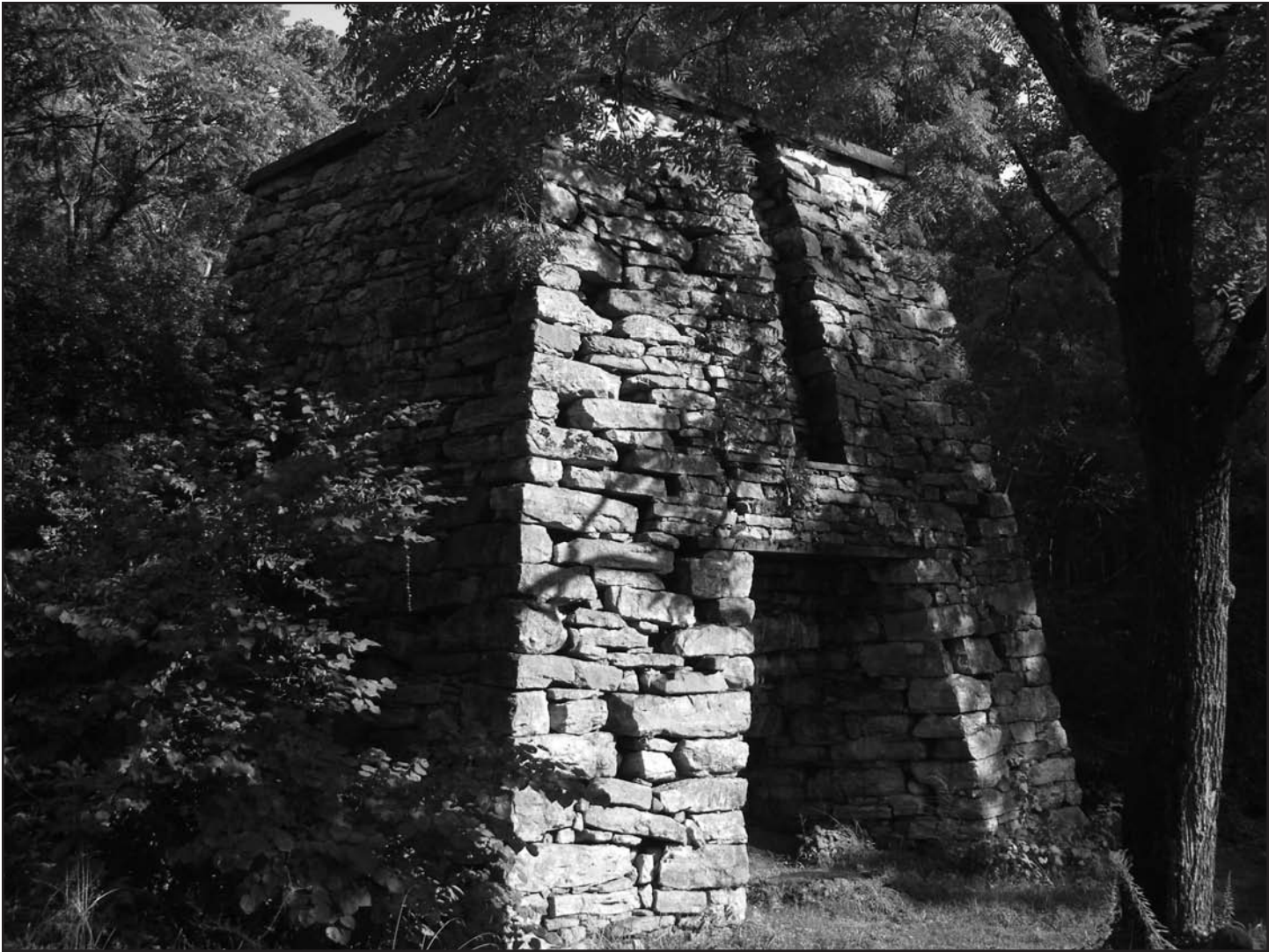
Figure 4.5. Catherine Furnace: the chimney for a 19th century iron furnace.
